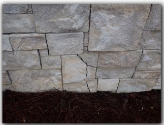
We observed some evidence of deteriorated mortar joints and cracking throughout the block exteriors of the entrance monuments at the Deer Creek Blvd property entrance. Refer to the following photos.
