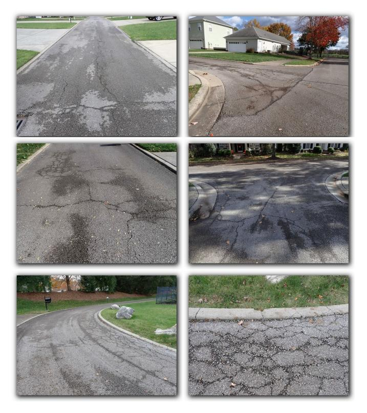
We observed some evidence of cracking and surface deterioration throughout the private, asphalt-paved road and parking area that serves the swimming pool area. Refer to the following photos.
