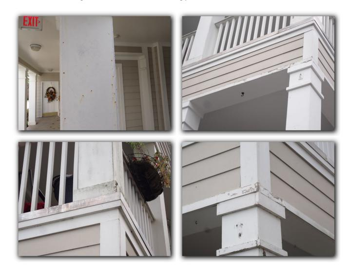
We observed general signs of deteriorated sealant throughout the fiber cement exteriors of the condominium building. Refer to the following photos.
