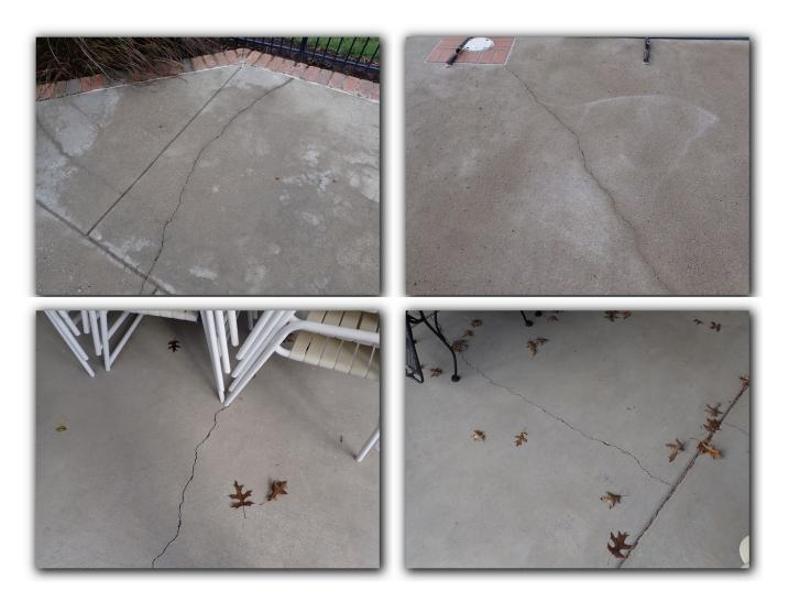
We observed general signs of deteriorated sealant between the concrete swimming pool deck and brick perimeters. Refer to the following photos.
