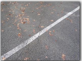
We observed evidence of deteriorated and fading parking space markings at the swimming pool parking area. Refer to the following photo.
