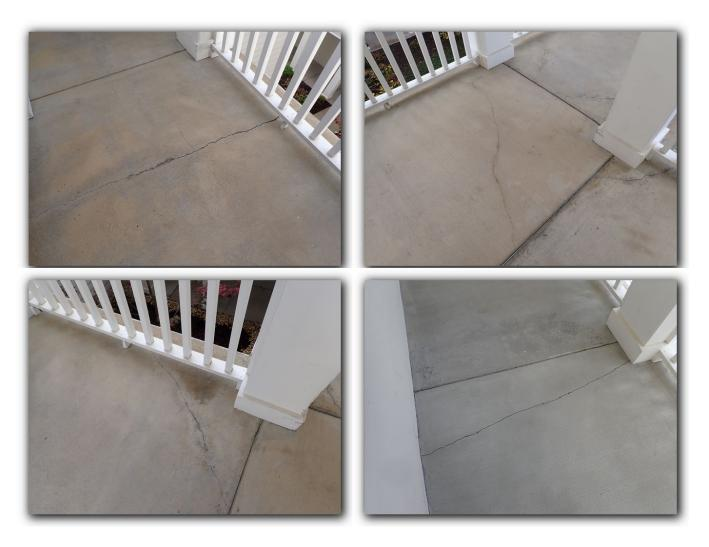
We observed general signs of surface deterioration throughout the uncovered concrete walkways around the condominium building. Refer to the following photos.
