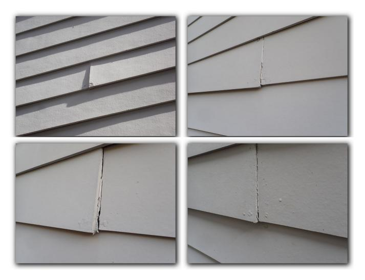
We observed some sections of damaged fiber cement siding near the bottom exteriors of the condominium building. Refer to the following photos.
